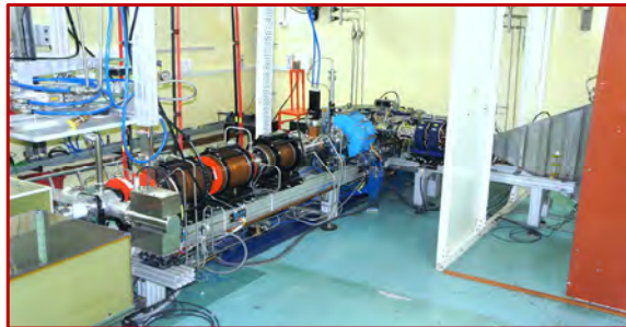
Linac-4 on test bench at RRCAT, 10 MeV, 15 kW
