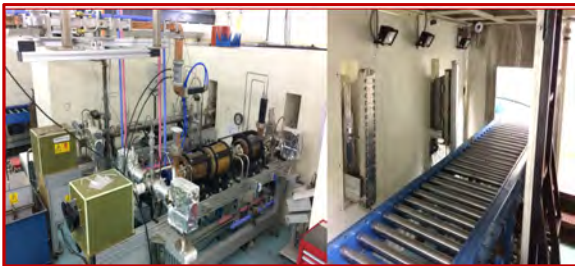
Linac-1 and Linac-2 (10 MeV, 6 kW) deployed at ARP
